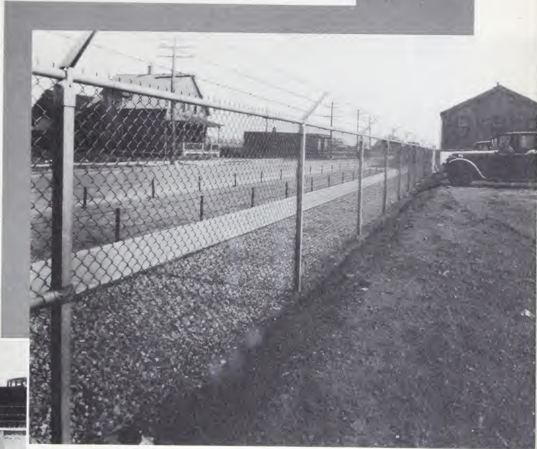
Above is a Cyclone Invincible Fence surrounding a parking yard. The name INVINCIBLE is clearly understood by a glance at the top of it . . . the arms along which barb-wire is strung. This fence is clearly impassable by any ordinary means and is largely used to enclose factory yards and industrial plants generally.
